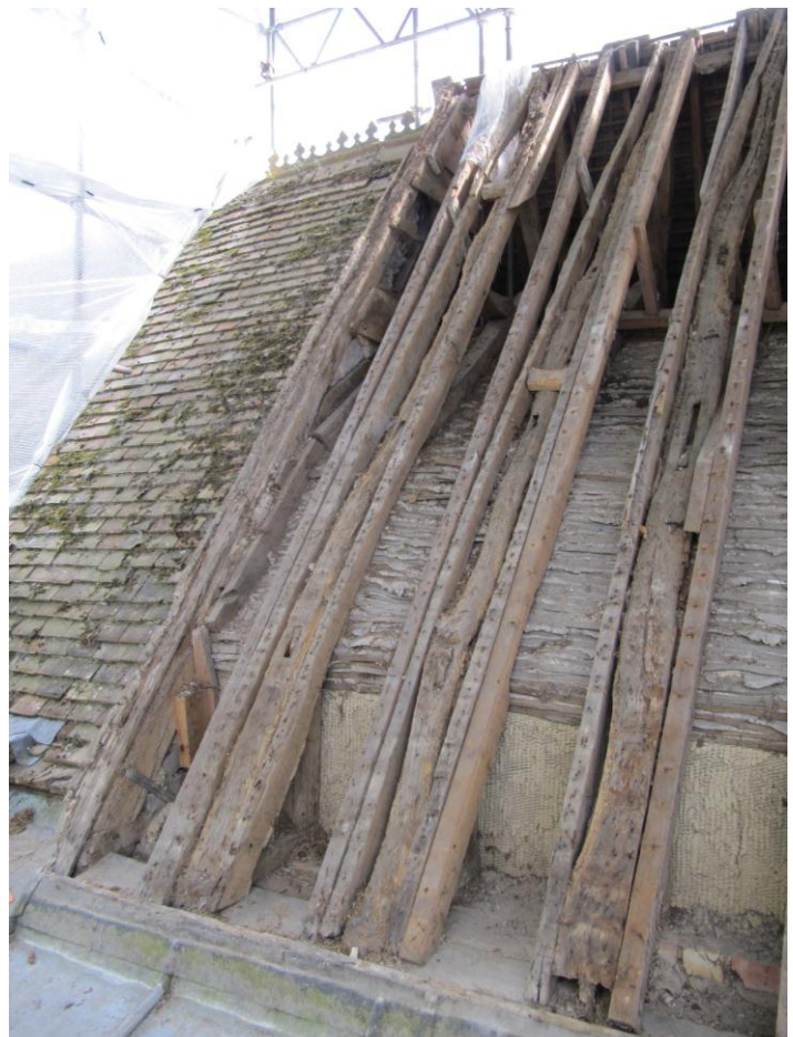
[Church of All Saints' Grafham. Nave Roof (North Slope). Note all previous partnering timbers]
