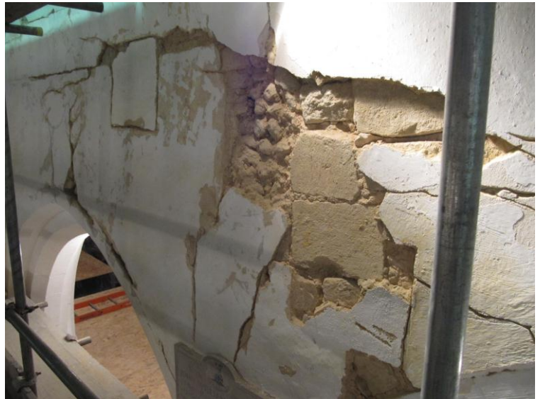
[Church of All Saints' Grafham. Nave (North Wall). Note structural movement]
