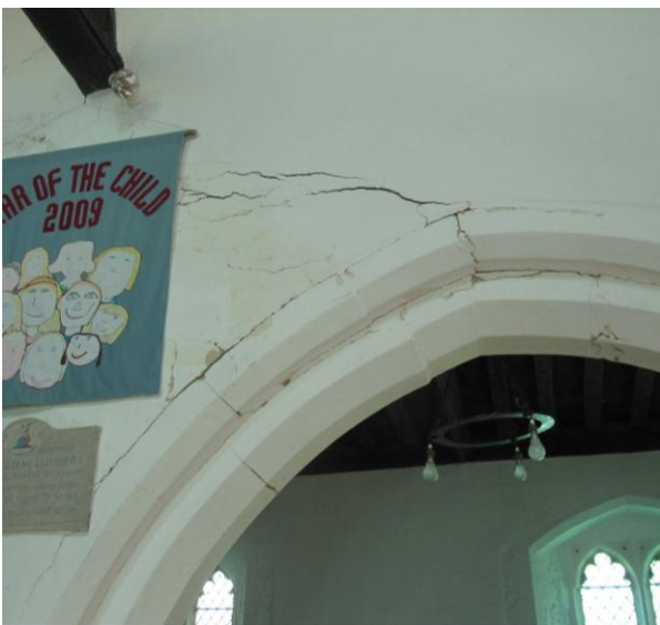
[Church of All Saints' Grafham. Nave (North Wall). Note structural movement]
