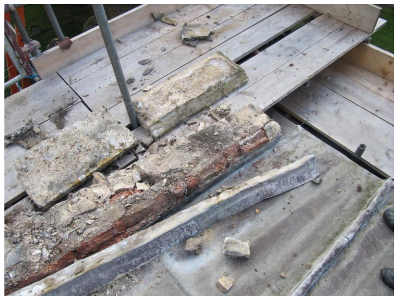
[Church of All Saints' Grafham. South Aisle Roof (East End) Location of parapet wall repairs.]
